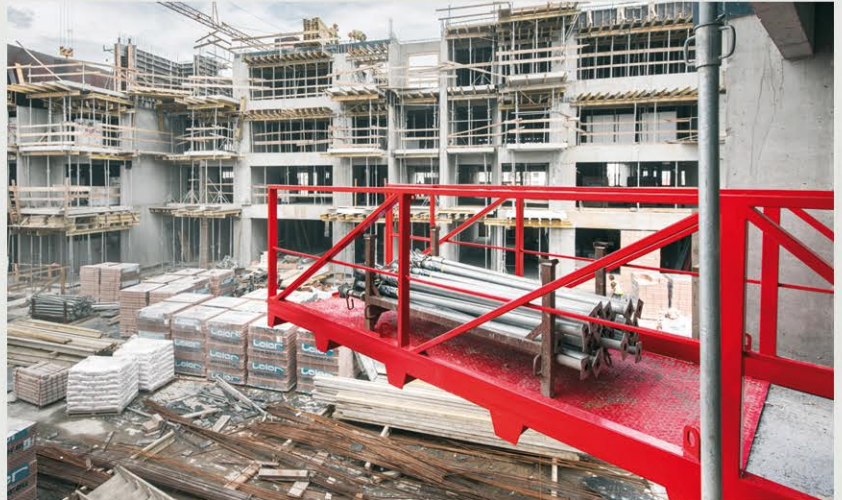
Carrying capacity of 4 tonnes, the platform's floor at the same level as the ceiling ensures ergonomics.
